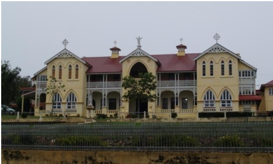
Mt St Bernard's College is an example of a Local Heritage place at Schedule 7 of the planning scheme.
